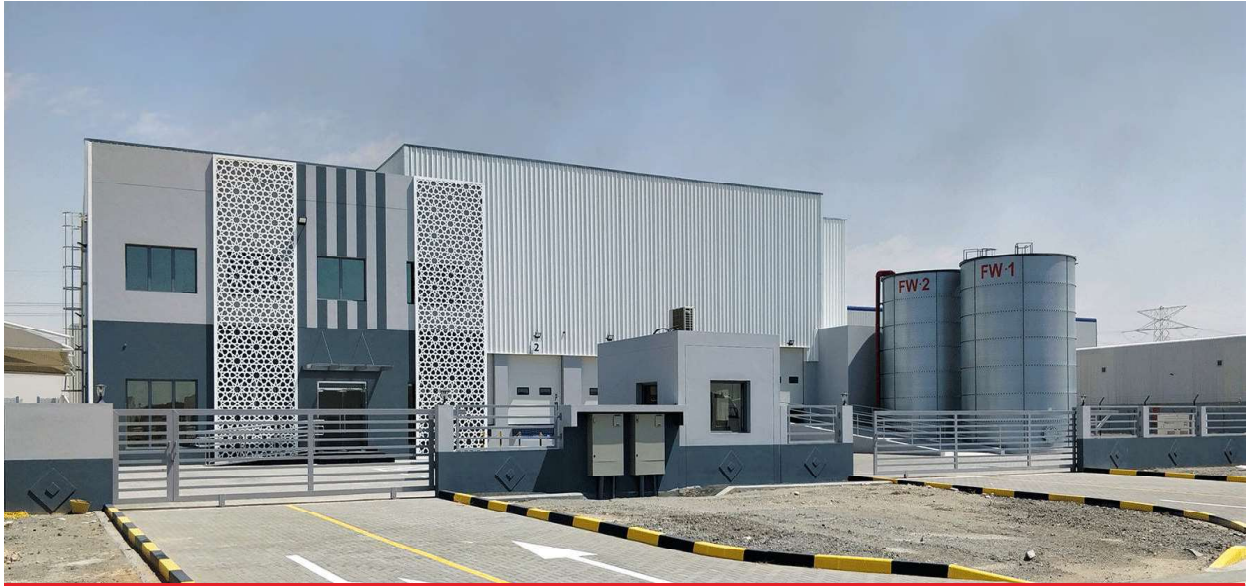
GRC CLADDING | WAREHOUSE | DUBAI - JABAL ALI
